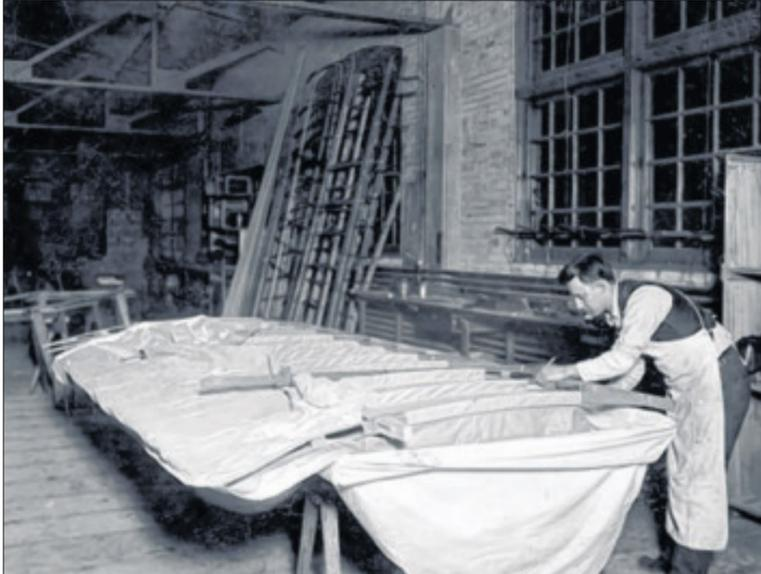
A worker applies fabric to an airplane wing in the original Wright Factory in west Dayton.
